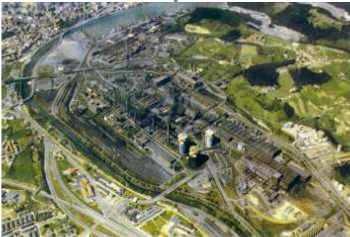
Ensidesa instalations before demolition, 1999.
